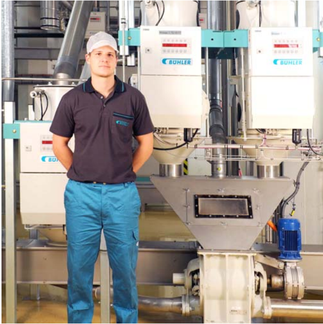
Buhler Scale Installation
