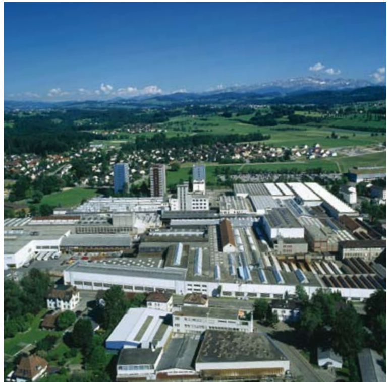
Corporate headquarters in Uzwil with production facilities and training centres.
